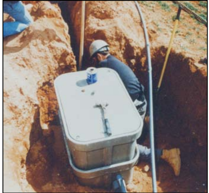
QUAZITE® enclosures are used for underground fiber optics and electric cable.
